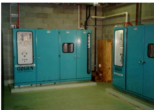
Figure 37 Corona discharge ozone generators
